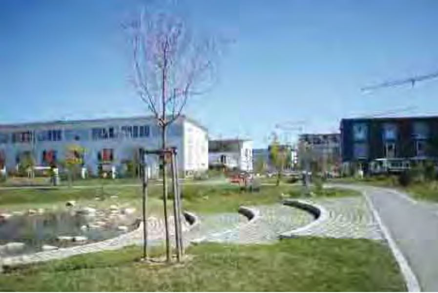
Figure 2.4 An example of a sustainable drainage system.
