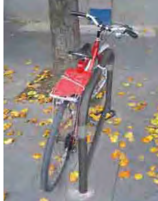
Figure 8.3 Sheffield stands are simple and effective. The design allows the bicycle frame and wheels to be easily locked to the stand. Note the tapping rail near ground level and the reflective bands on the uprights.
